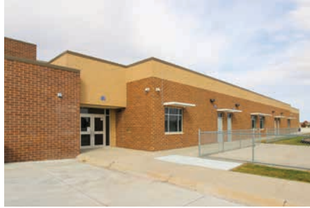
Shoemaker Elementary Classroom Addition
