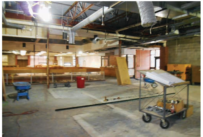
The Campus Center after demolition work.
